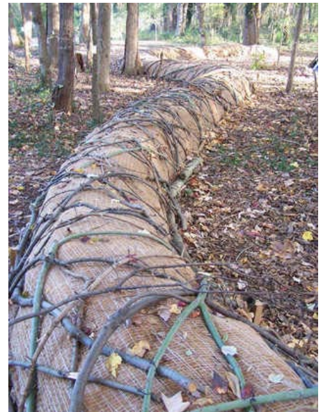
Twig-covered tubes of brush and other natural materials are designed to slow and absorb rainwater runoff, protecting Little Sugar Creek from pollution.
