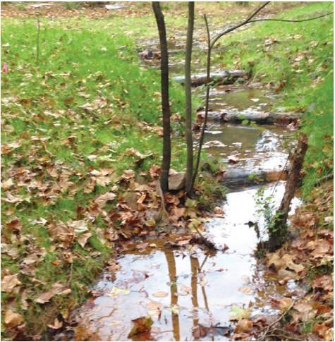
Logs were installed in the bog to help mimic natural sheet-flow of water.
