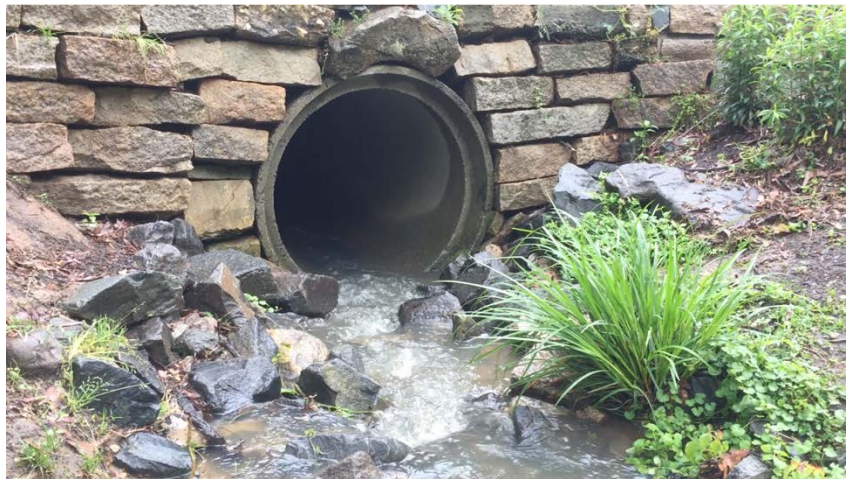
Water flowing into a culvert from a small tributary in Midwood Park
